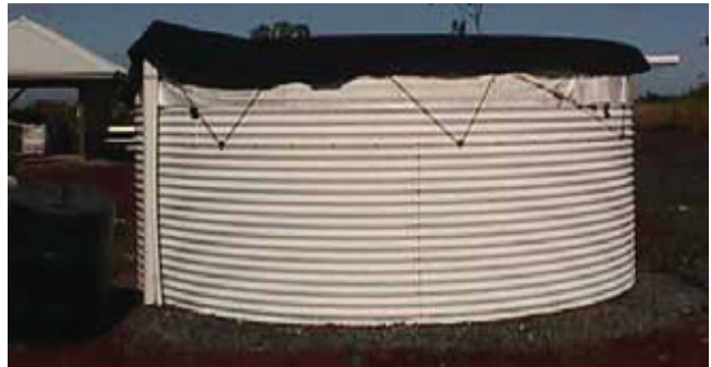
A typical corrugated steel tank with a mesh cover. This type of tank is the second most common in use today.
