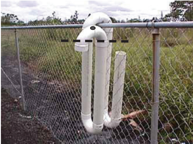
An overflow device to keep the water level, as indicated by the dashed line. Pipe on the near side of the fence hangs outside the tank. A hole atop the elbow in the foreground is needed to break the siphon so pipes will remain primed with water for the next rainfall event. A T-joint could be used instead of an elbow with a hole.
