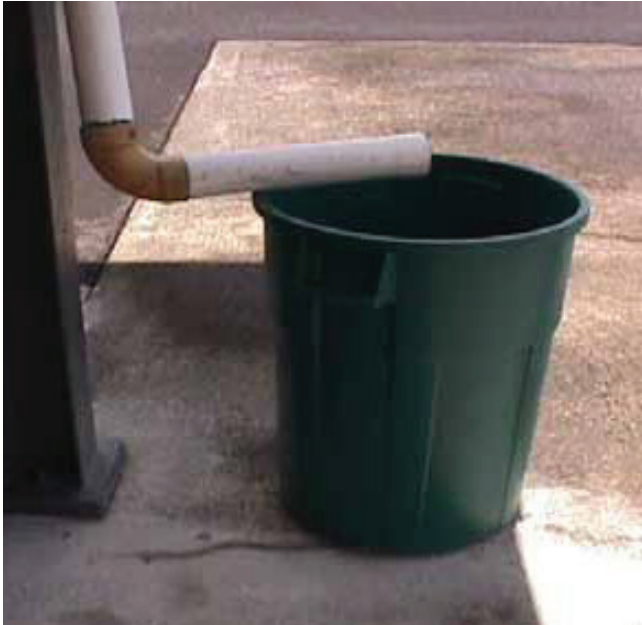
Water collected and held in containers that haven't been approved for water storage can be deadly. Plastic garbage containers, for example, can contain toxic dyes and biocides that could leach into the water.
