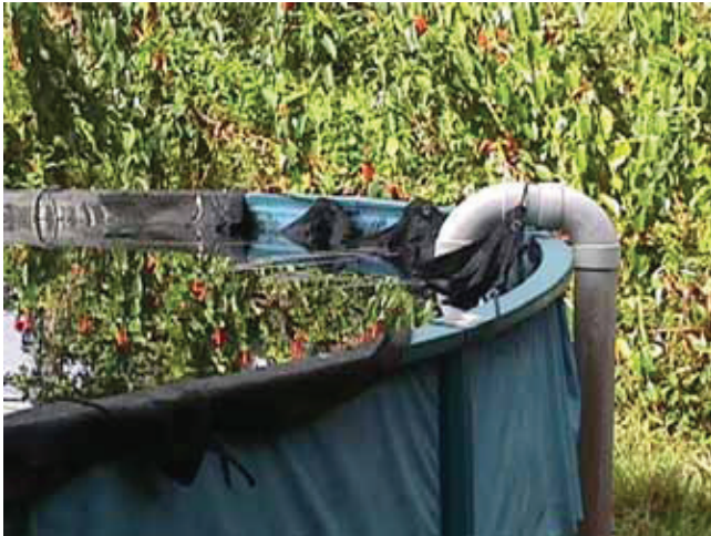
Sagging and broken covers like this one are very common. The storage tank is where water sits the longest, and keeping it covered is important to reducing water contamination.
