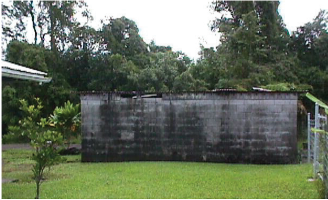
Hollow tile tanks have lost popularity mainly due to their price and tendency to leak.
