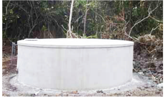
Ferroconcrete tanks, also known as ferrocement tanks, are new to the local market and growing in popularity. Like solid concrete tanks, they can be designed into a home's structure.
