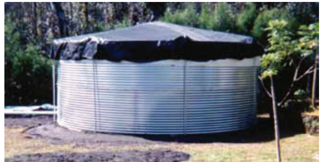
Pipe arches supporting a mesh cover keep it from sagging into the water.
