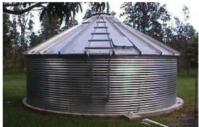
Some corrugated tanks have solid covers. This model has a top hatch for access and a liner secured to the sides with bolts.
