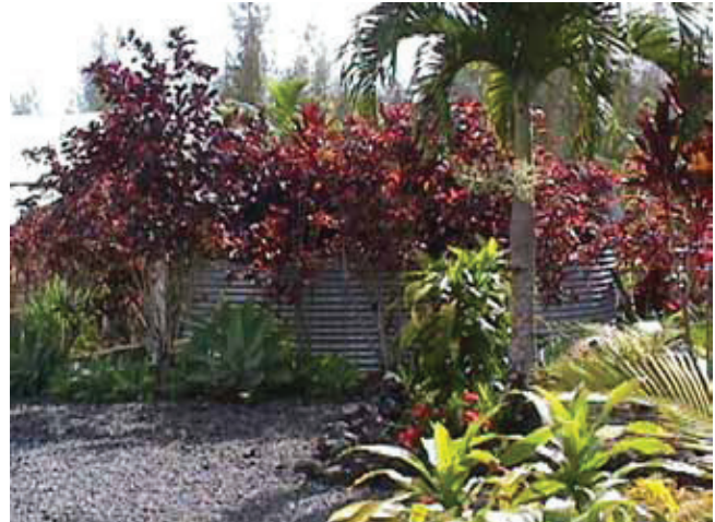
Even though surrounding your tank with plants may look nice, it can cause major pollution problems for your water supply, particularly if the tank cover is not solid.
