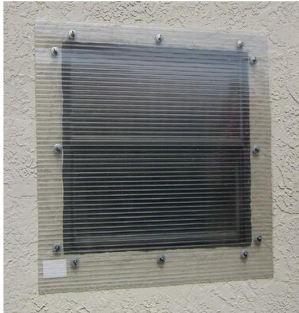
Polycarbonate storm panel installed with wingnuts and washer attached to permanently installed threaded studs.
