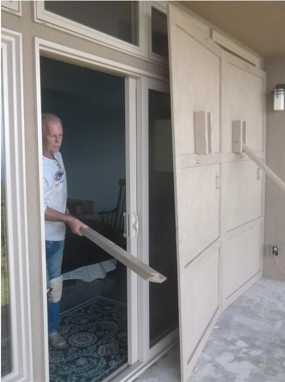
Rather than use fasteners, this homeowner is using wooden braces to keep the panels in place.
