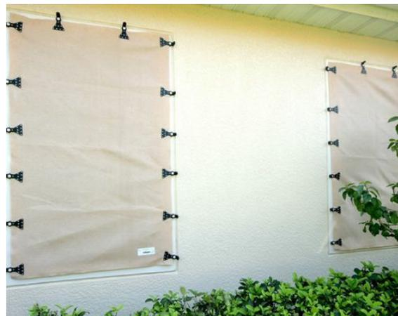
Heavy plastic clips are permanently attached to the fabric. Permanently installed fasteners around the opening go through the clips.
