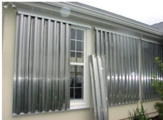
Corrugated aluminum storm panels in tracks. They can also be installed with individual hardware permanently
